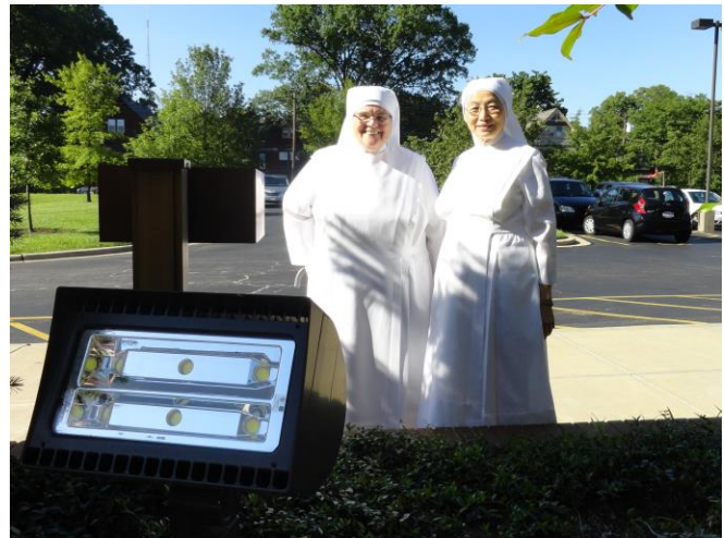
Sr. Katherine Ann and Sr. Dora with one of the new LED lights already installed to test performance.
